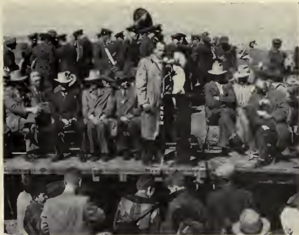
AT VERMEJO CELEBRATION, sponsored by the Directors of the Vermejo Conservancy District, E. D. Eaton, Director of Reclamation's Operation and Maintenance Division addresses the crowd on the site of old Stubblefield Dam. Photo by F. S. Finch, Region 5.
